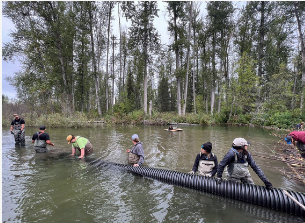
Installing a pond leveler as a beaver co-existence strategy
