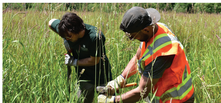
NCC work-pod installing live stakes at Chase Woods Nature Preserve. Photo by Wetlands Workforce.
