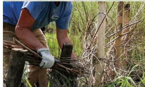
Schematic for a BDA (left, Wheaton et al. 2019). BDA construction using a post-pounder and a vegetation weave (right, Koenigsberg 2018).
